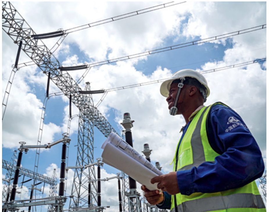
A local worker is pictured at the Konza transformer substation being built by a Chinese company in Machakos County, Kenya, on 5 May
